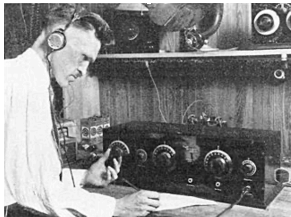
Figure 31 TRF Receiver (source:Wikipedia)
